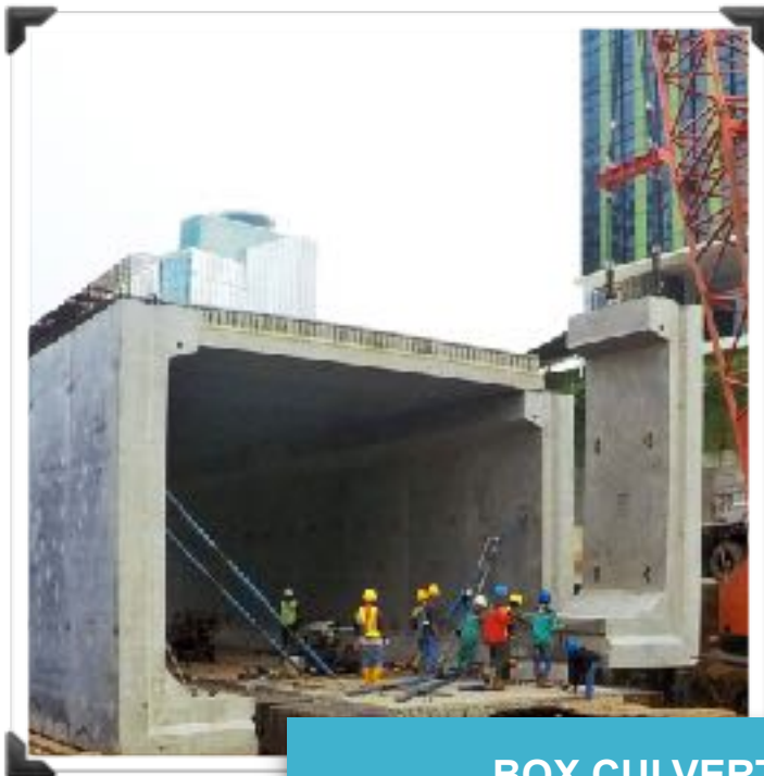
BOX CULVERT DEPOK-ANTASARI TOLL ROAD
