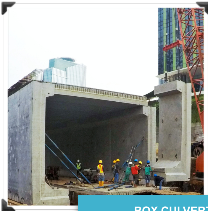
BOX CULVERT DEPOK-ANTASARI TOLL ROAD
