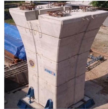
PIER PRECAST SEGMENTAL
