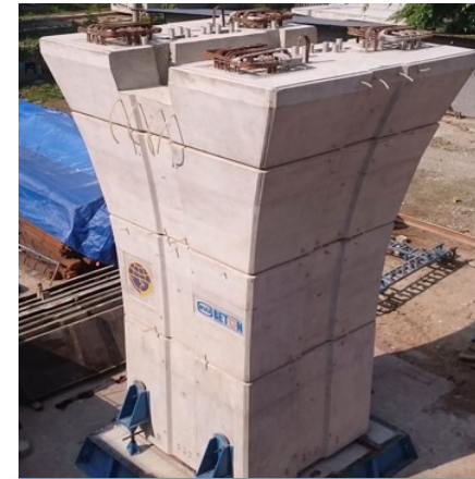
PIER PRECAST SEGMENTAL
