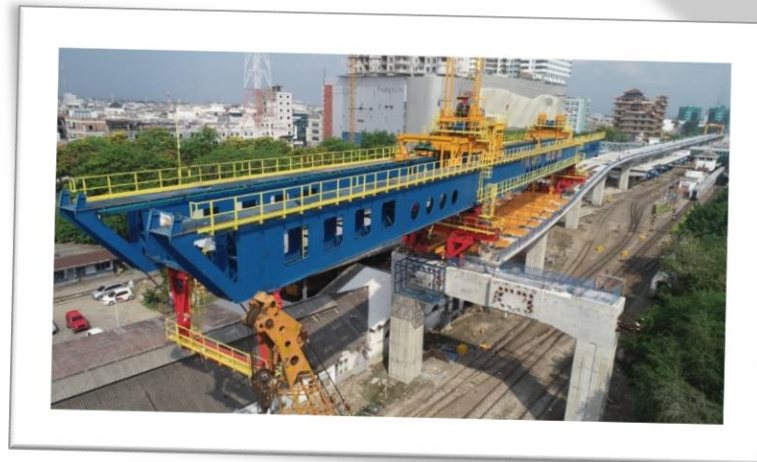
LAUNCHING GANTRY: 11 LAUNCHING GANTRIES
