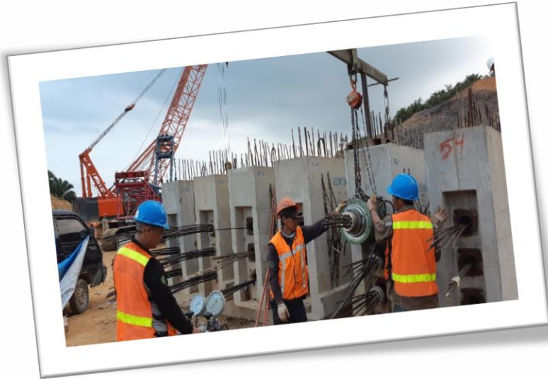
POST-TENSIONING: 84 POST-TENSION TOOLS
