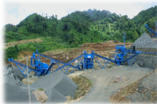
QUARRY & CRUSHING PLANT
