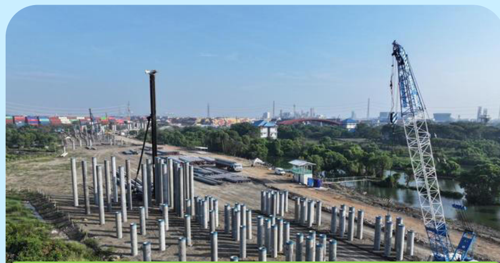
New Priok East Access
